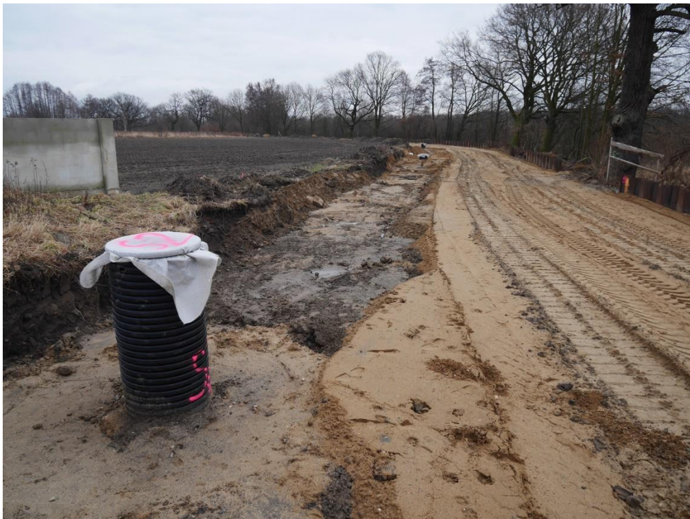
Phot.4. Drainage along the constructed flood protection embankment in the first implementation section, along avenue of oaks no. 28 – Task 1
