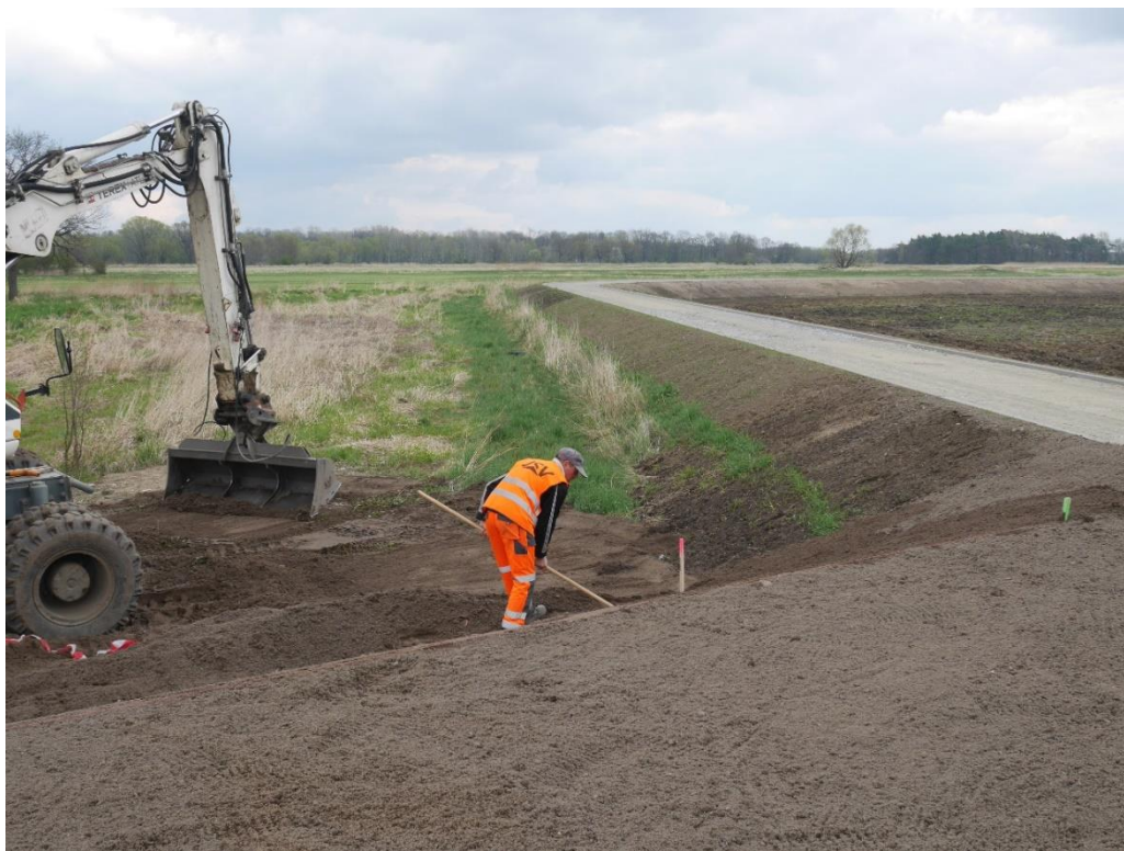
Phot. 51. Topsoiling of flood protection embankments – Task 5
