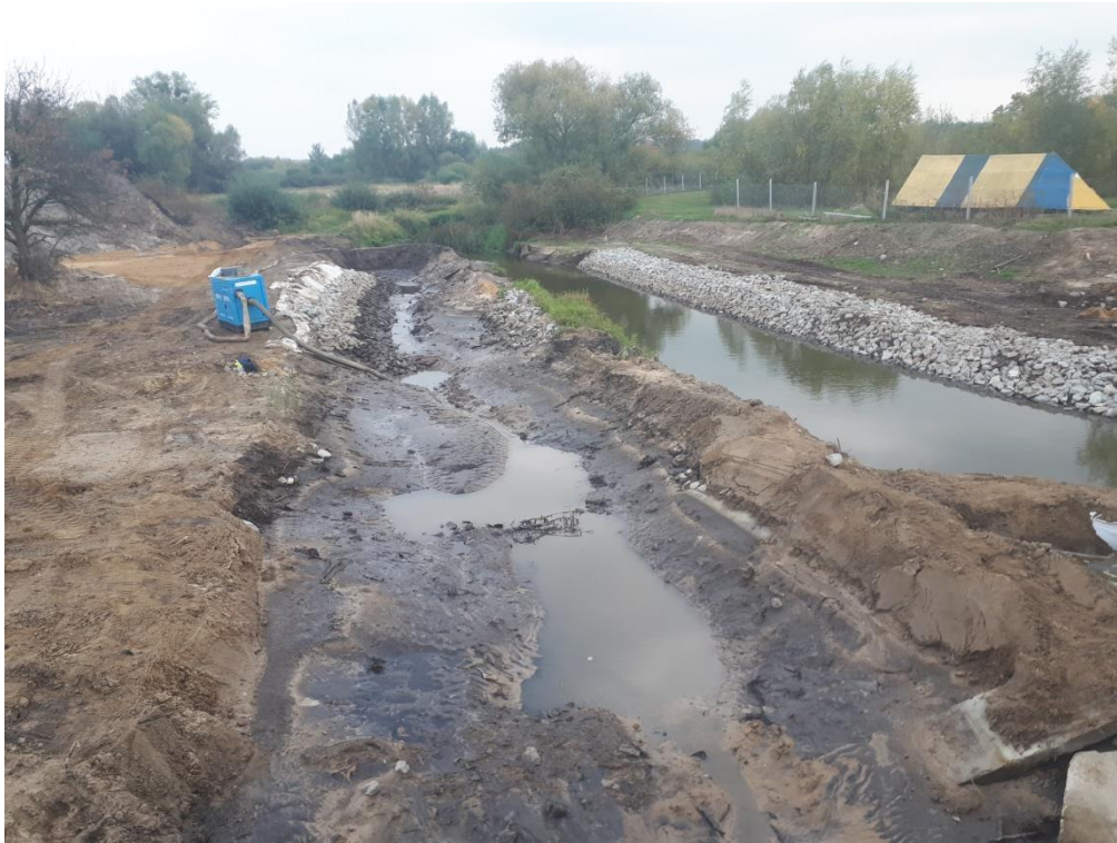
Phot.7. Water pumping from desludged section of the Widawa upstream of the bridge at Rieczna Street – Task 1
