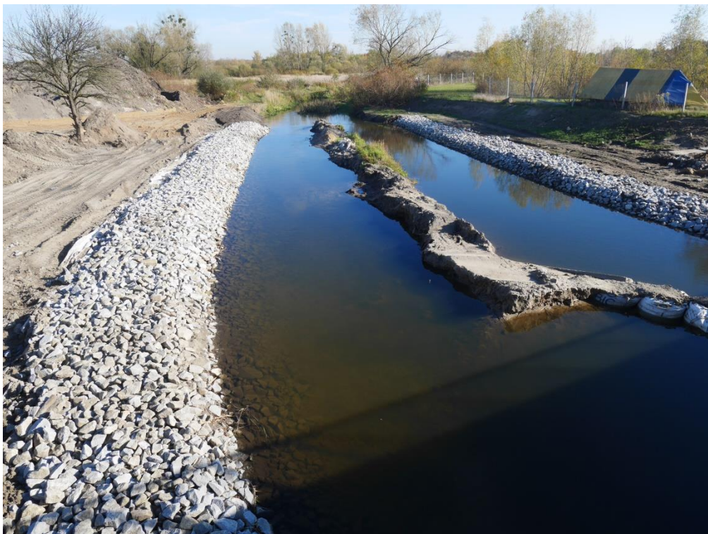
Phot.8. Regulation works at the Widawa, upstream of the bridge at Rieczna Street – Task 1
