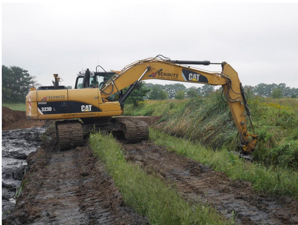
Phot.44. Desludging of the ditch R-G, carried out under nature supervision – Task 4
