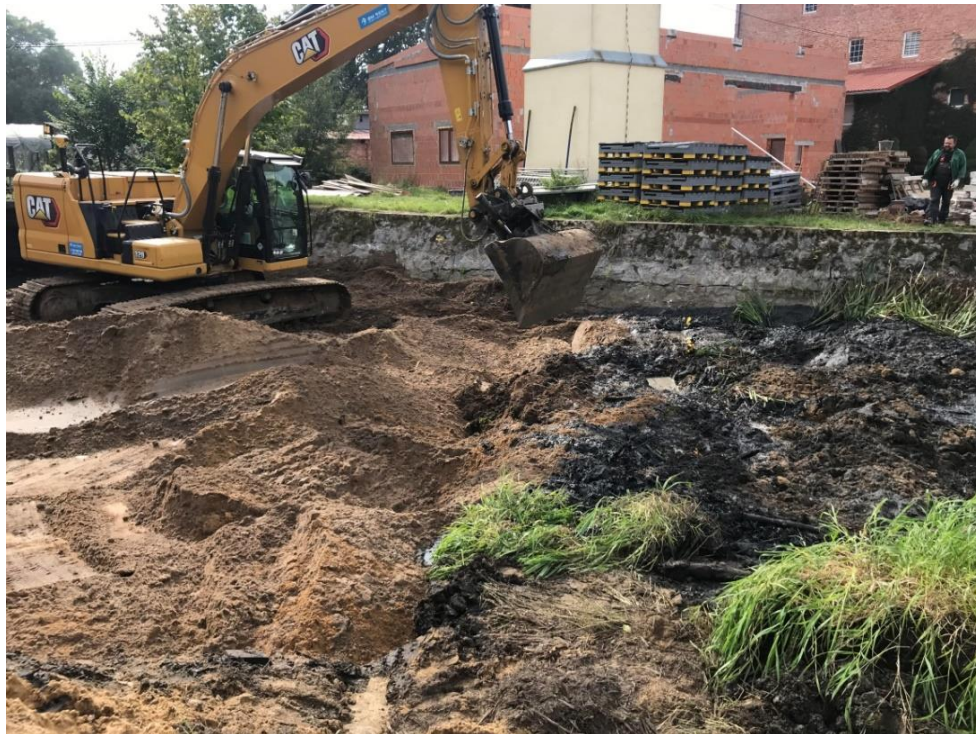
Phot.32. Removal of the old, estuary section of the Młynówka Kielczowska bed – Task 3
