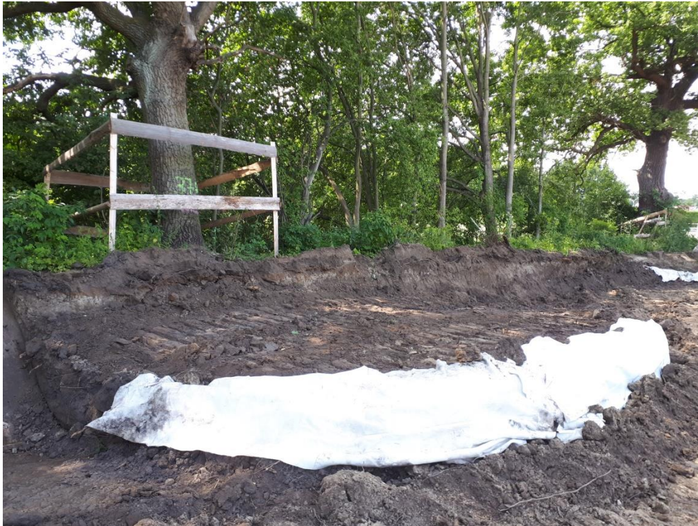
Phot.1. Roots of oak trees at natural site no. 28 secured from drying out, after topsoil removal – Task 1
