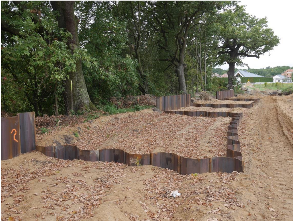
Phot.3. Bypasses of oak tree roots constructed using sheet pile walls at natural site no. 28 – Task 1
