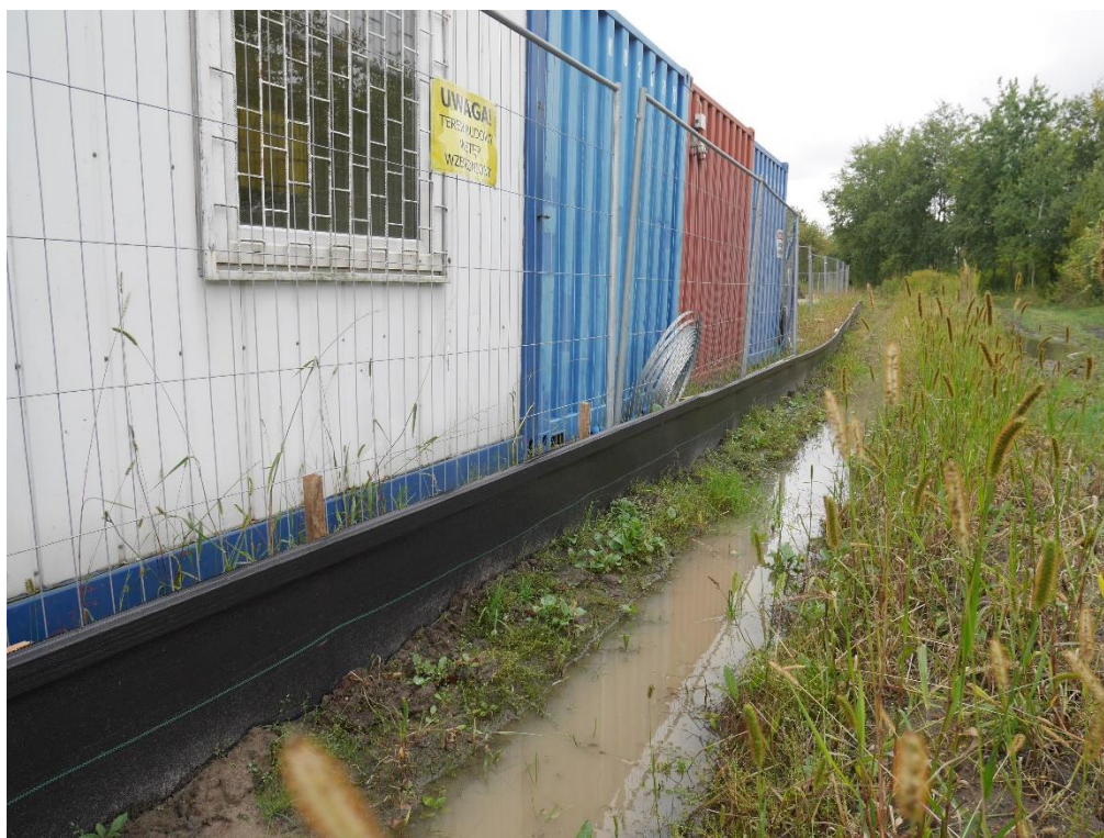
Phot.43. Herpetological fence around the construction in September 2020 – Task 4
